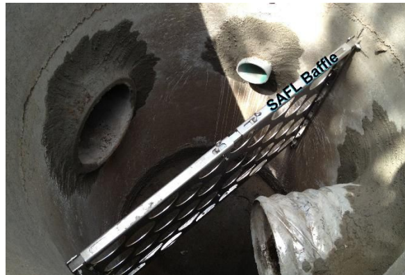
The SAFL Baffle from Upstream Technologies, Inc. helps cities treat urban runoff that goes into storm sewers and eventually ends up in lakes, rivers and oceans.
